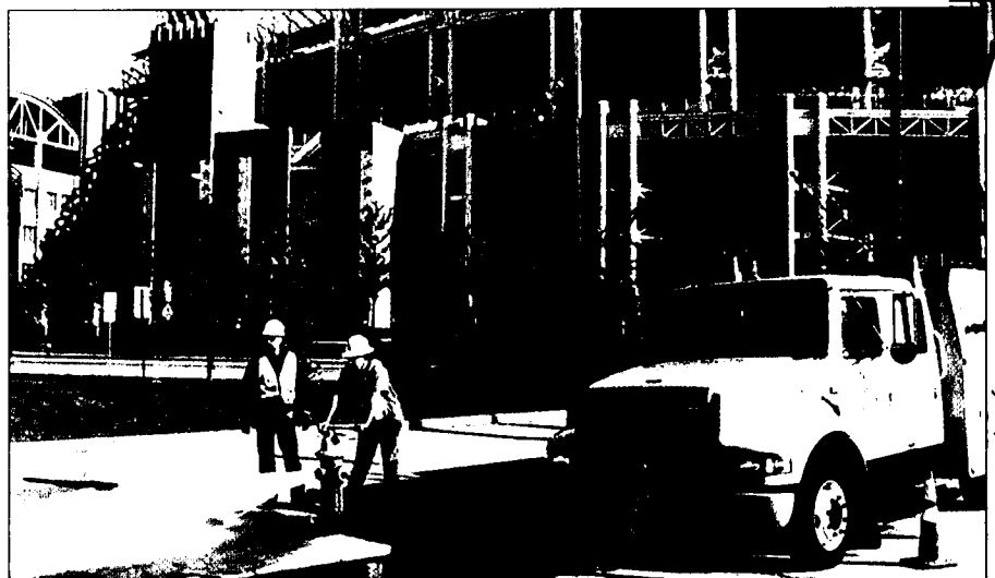
Maintaining critical infrastructure components, such as flushing hydrants, is a key component of a utility's operations and maintenance program.
